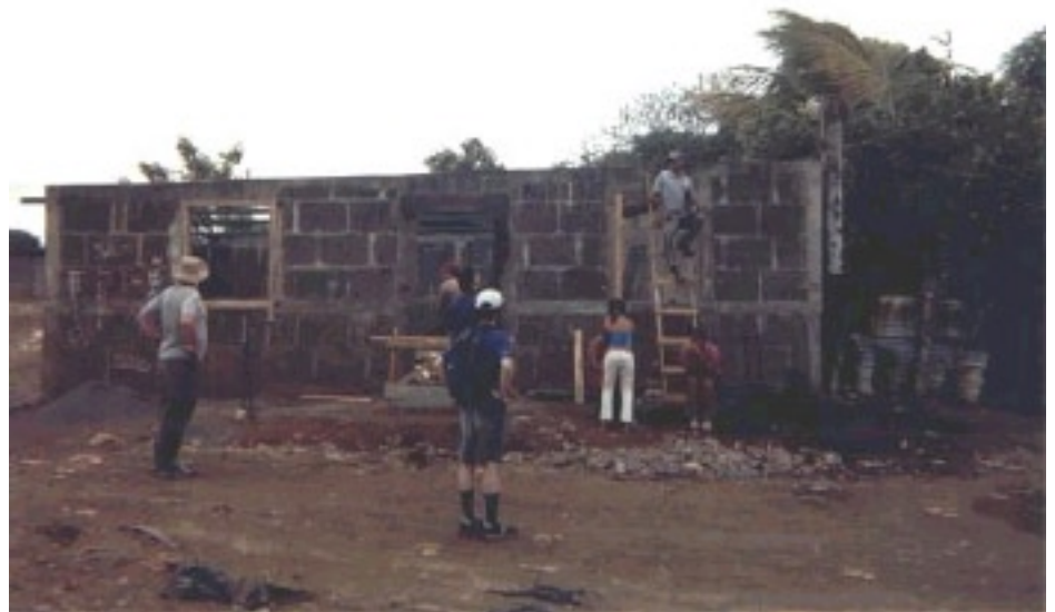
The new WIA building.
