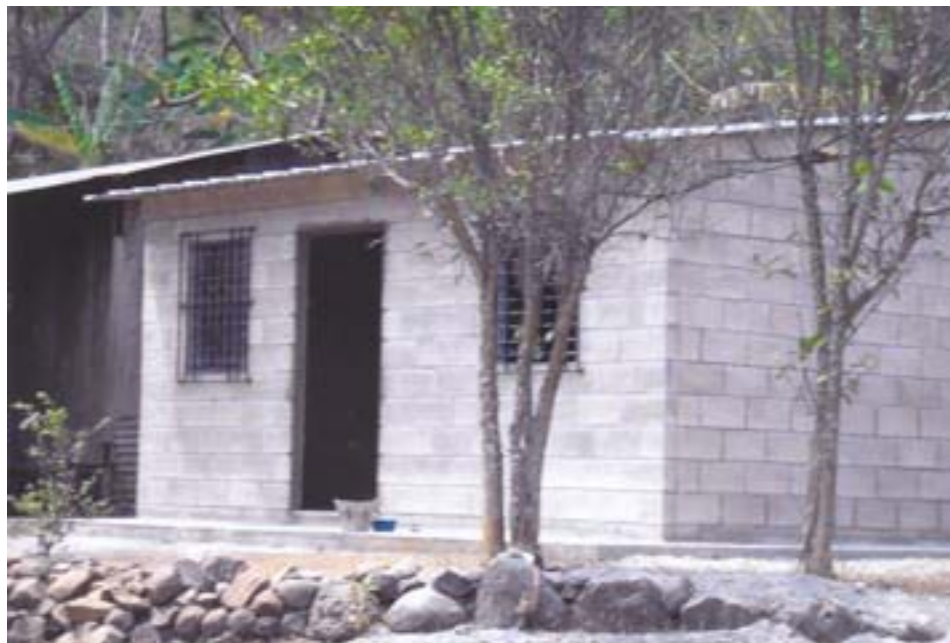
One of ten recent Habitat for Humanity homes built in Valle Nuevo.
