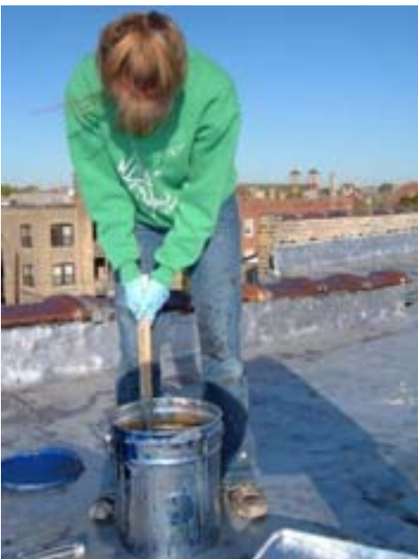
Hope mixing the roofing cement.
