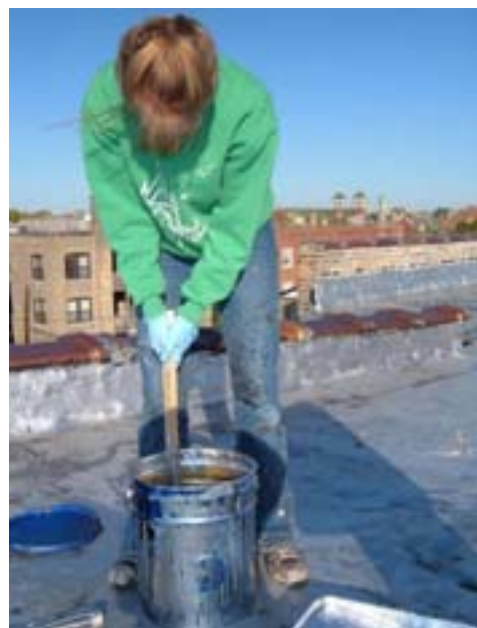
Hope mixing the roofing cement.
