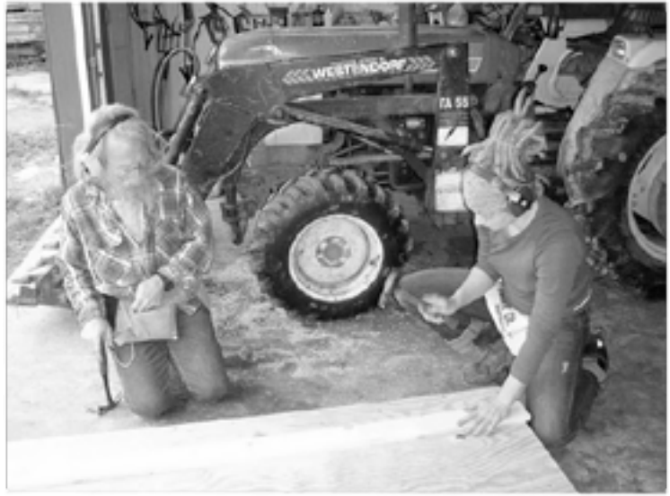
Jim Foxvog and Emily Adama work together on building the privy
